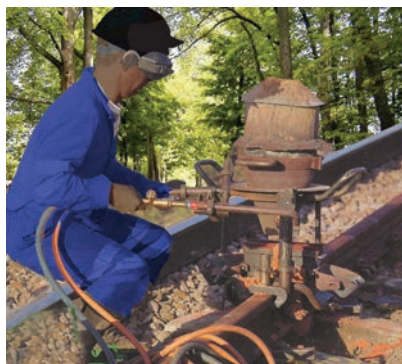
Figure 3.11 Thermit process for joining railway tracks
